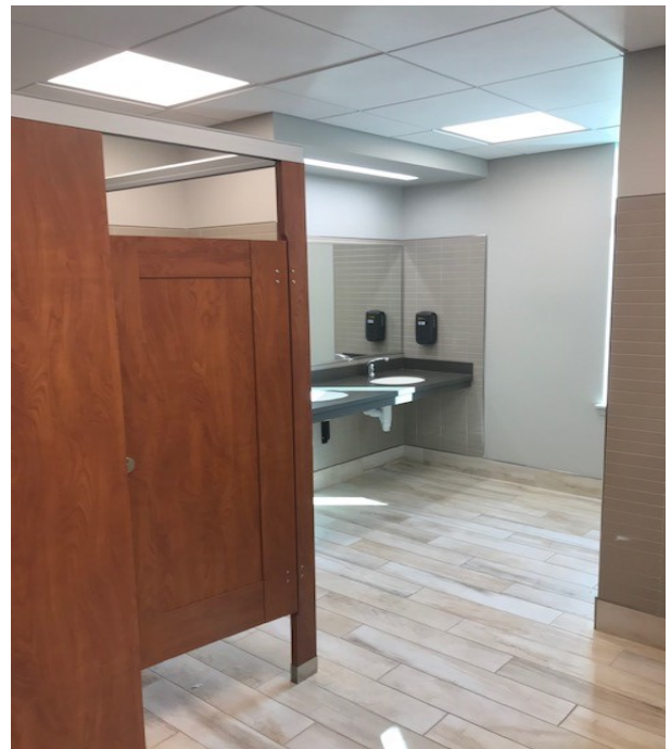
Newly renovated restrooms
